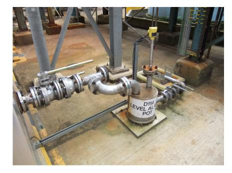
Moisture detection pot with resonant type detector with alarms
